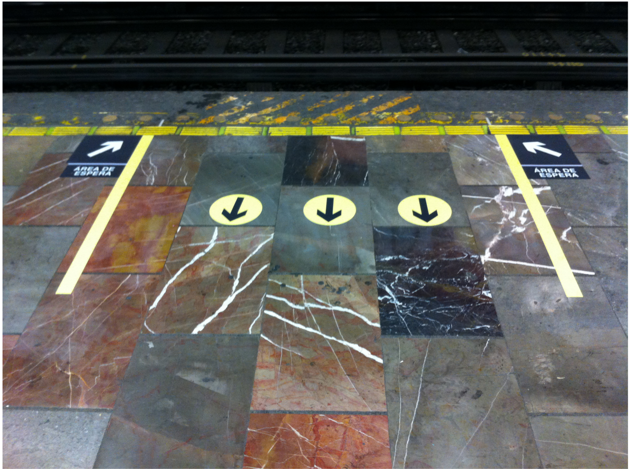
Fig 15. Guide sign on the platform. The components of the guide signs are: three circles that indicate the way to exit, two vertical lines dividing the waiting area, and two black boxes with sideline arrows to indicate the boarding orientation.
